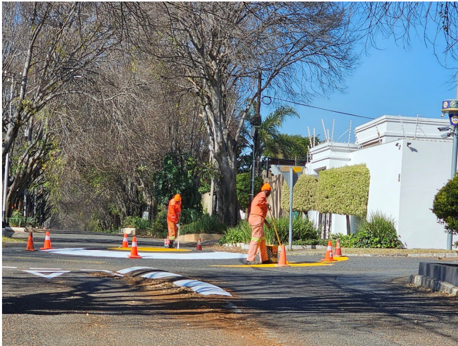
Road marking painting underway, 15 th July 2025
