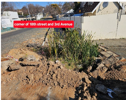
Reinstatement in Road. Corner 18th St. and 3rd Ave. Parkhurst. Ref # 5465792
